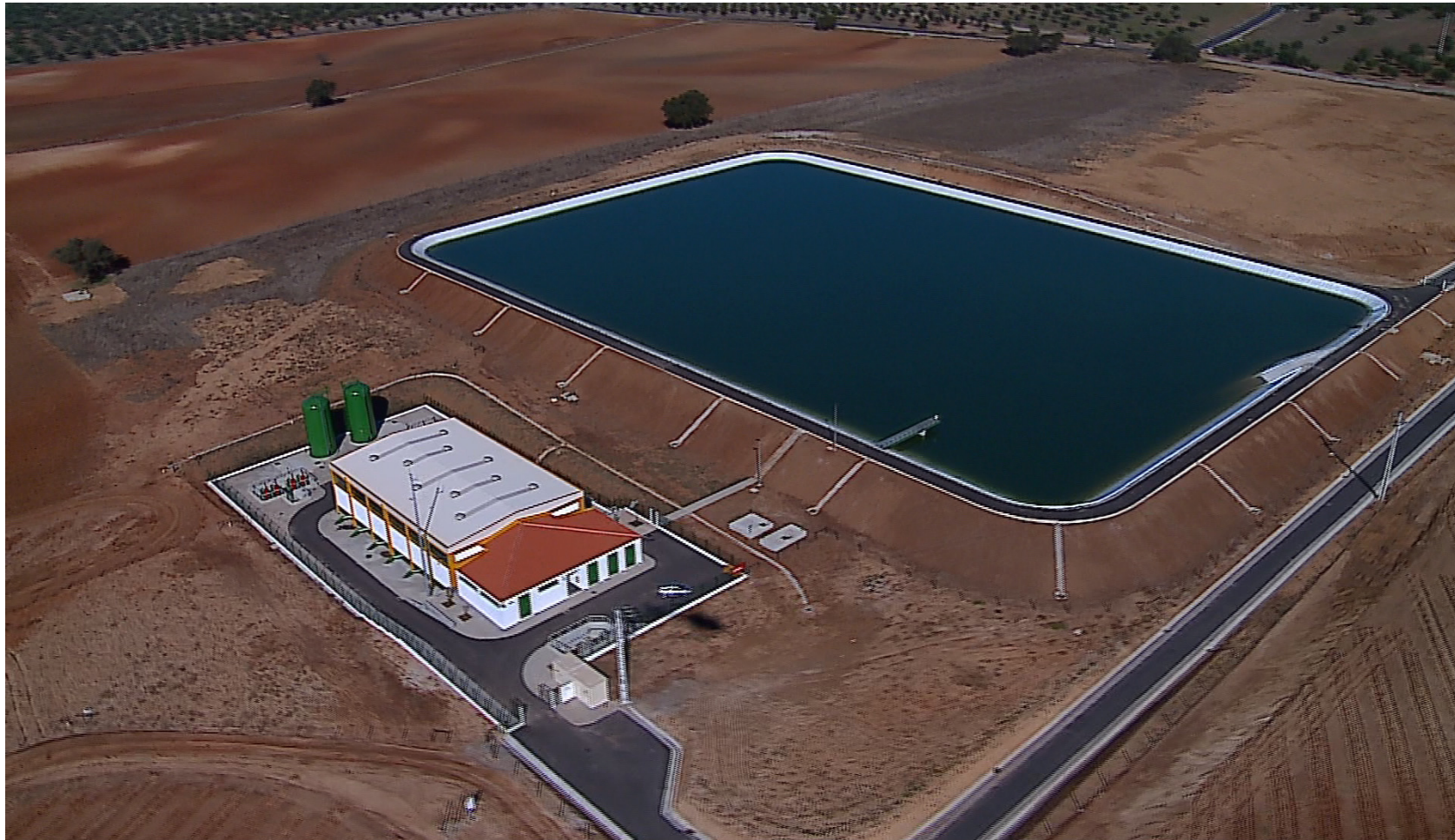
RESERVOIR AND SECONDARY PUMPING STATION
